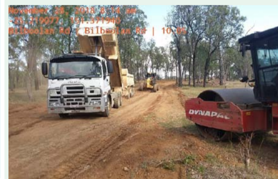
Bilboolan Rd Restoration works, Mount Perry under construction.
