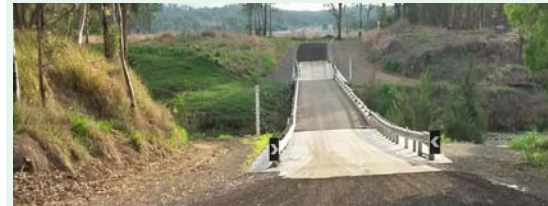
Waratah Bridge on Cahalane Road, Monto (Completed NDRRA project).
