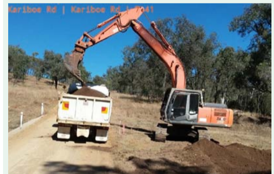
Kariboe Rd, Monto 'under construction'.
