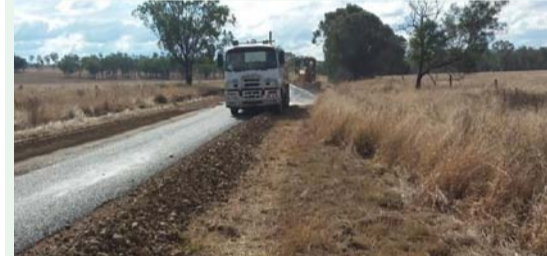
Abercorn Rd, Eidsvold 'under construction'.
