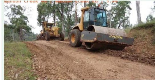
Mahoon Creek Rd, Monto 'under construction'.
