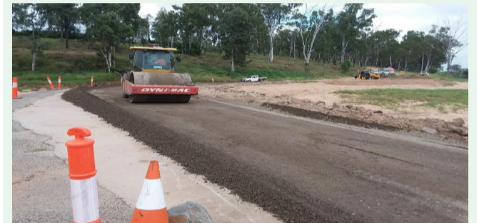
Yenda Benyenda Rd, Gayndah 'under construction'.
