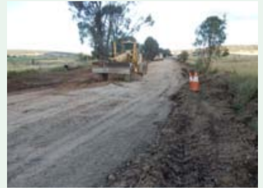
Church Rd, Mundubbera 'under construction'. This work is now complete.
