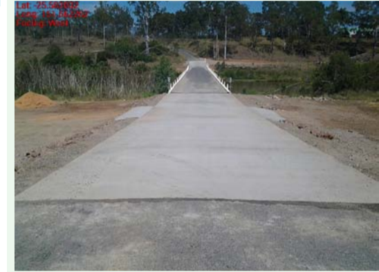
Bon Accord bridge approach, Gayndah.
