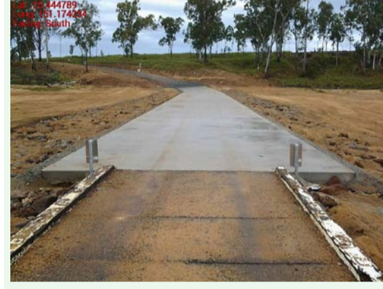
A Creek Rd, Mundubbera 'completed'
